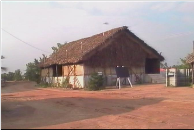
The rebuilt Yagashala
